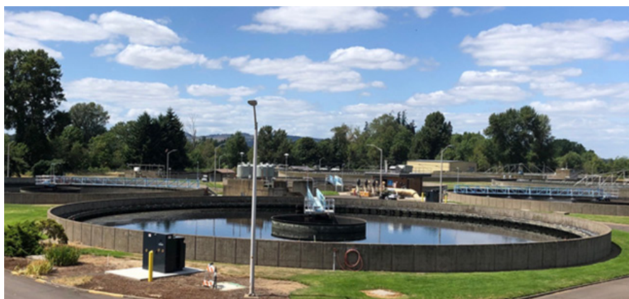
Secondary Clarifier at the Willow Lake Water Pollution Control Facility ▶
