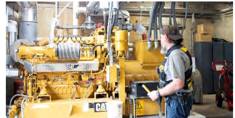
2023 – Biogas cogeneration engine at Tri-City WRRF
