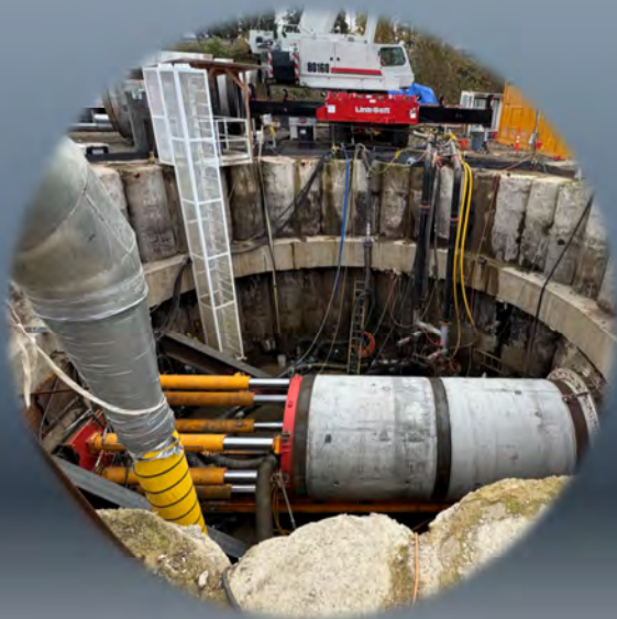
Sections of pipe are added as Clack-A-Mole continues digging the half-mile-long tunnel.
