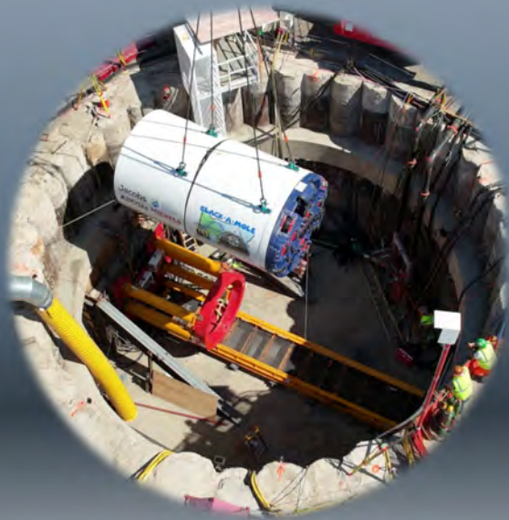
The tunnel boring machine “Clack-A-Mole” is lowered into the launch shaft.
