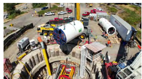
2024 – The “Clack-A-Mole” Tunnel Boring Machine is lowered into the launch shaft
