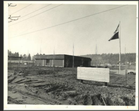
1974 - Construction of the Kellogg Creek Water Resource Recovery Facility (WRRF)
