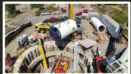
2024 – The “Clack-A-Mole” Tunnel Boring Machine is lowered into the launch shaft
