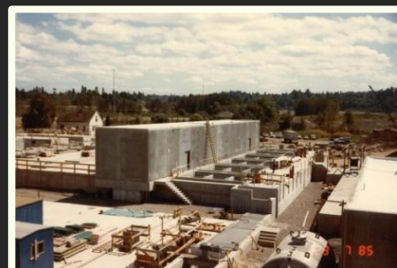
1985 - Construction of the Tri-City WRRF
