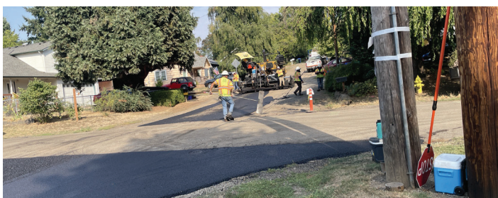
DOWL's inspectors monitored grinding and paving operations in 11 different neighborhoods across the City.
