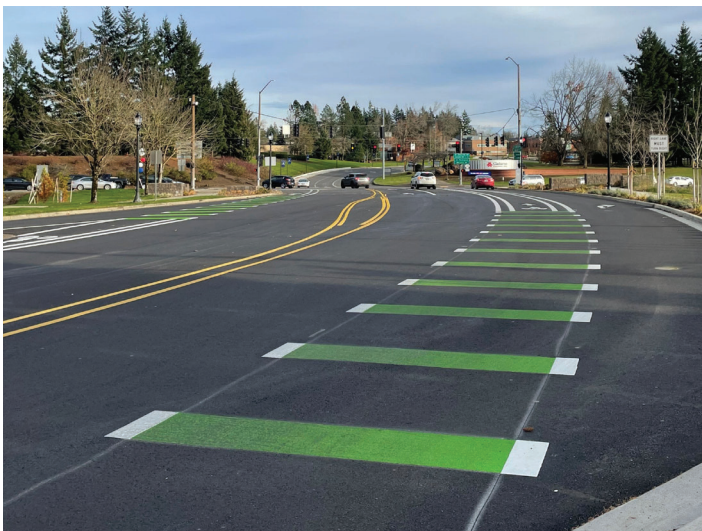
DOWL monitored inspection of full roadway reconstruction, storm improvement, and accessibility with new sidewalk and bike lanes.
