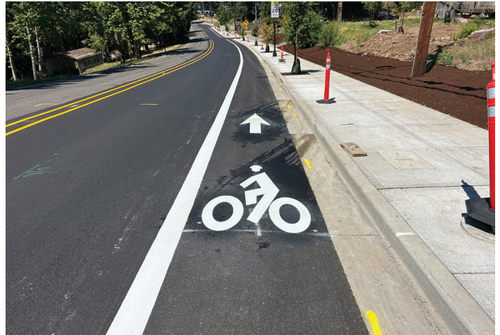
DOWL monitored inspections to improve accessibility to Holcomb Elementary School, including sidewalk, bike lane, and paved travel lane enhancements, along with updated roadway striping.
