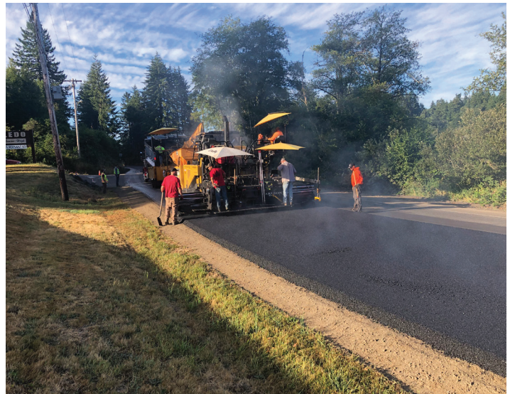
DOWL QCCS monitoring placement to make sure contractor performed the work as outlined in the contract.
