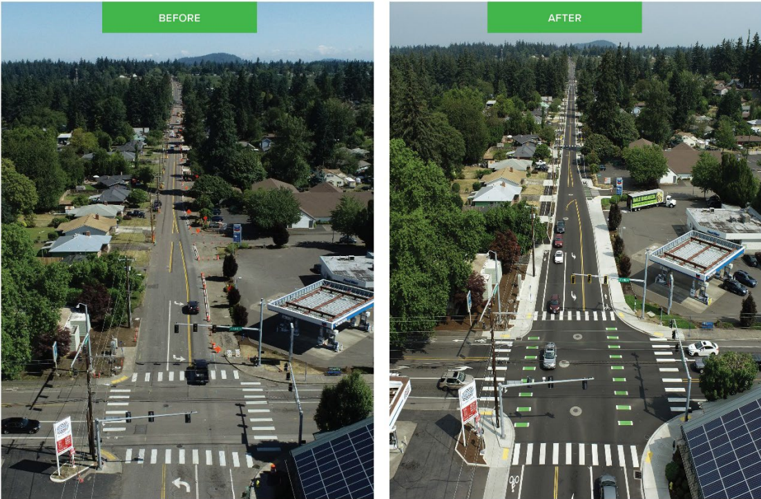
LINWOOD AVENUE IMPROVEMENT PROJECT >> CITY OF MILWAUKIE & CLACKAMAS COUNTY
