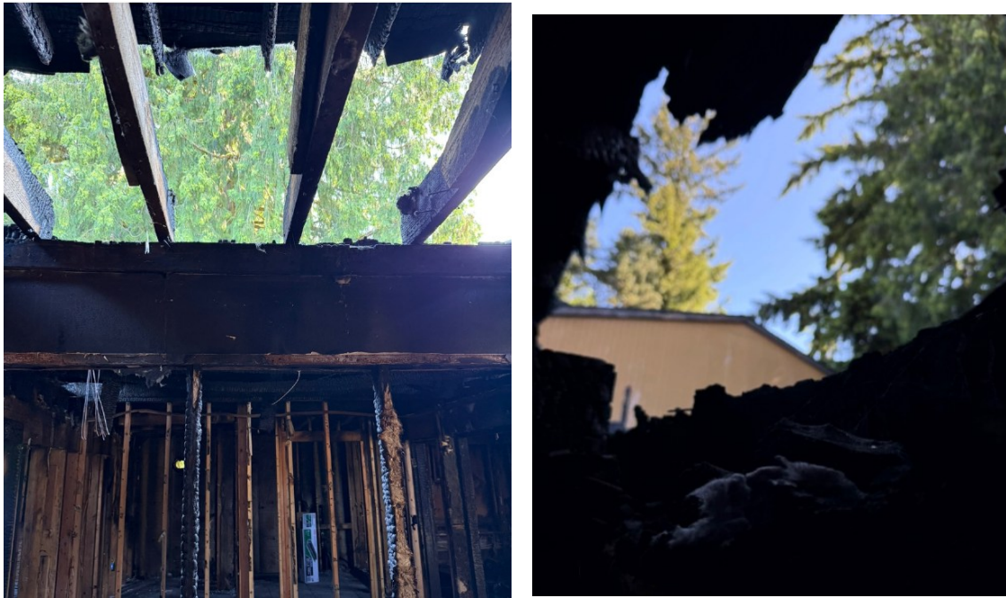
Figure 1 – Hole in the roof of the front portion of the building
