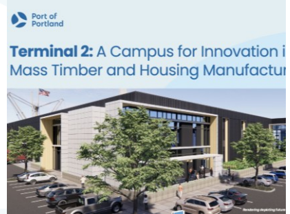
Mass Timber and Housing Innovation Campus at T2
