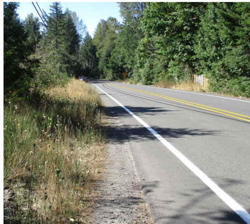
Lolo Pass Road Paving Overlay in Rural Environment
