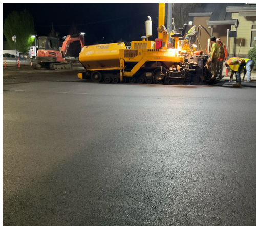
Paving Inspection for Clackamas County Night Inspection Services
