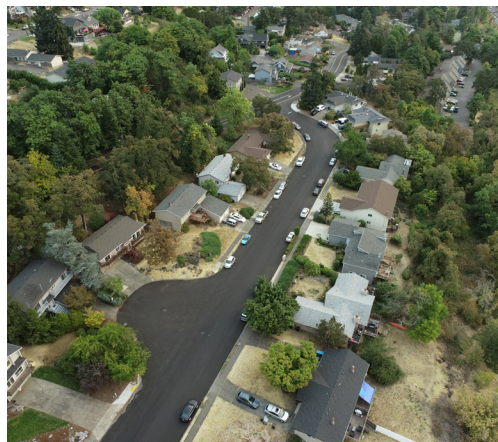
Residential Neighborhood Paving West Linn Road Program
