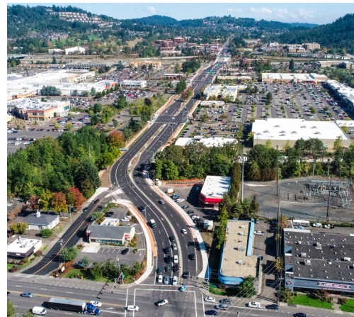
CRC Mobility Improvements Ramp and Pavement Construction Services
