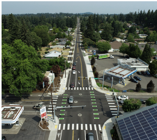
Linwood Avenue Improvements Pavement Rehabilitation Along Corridor
