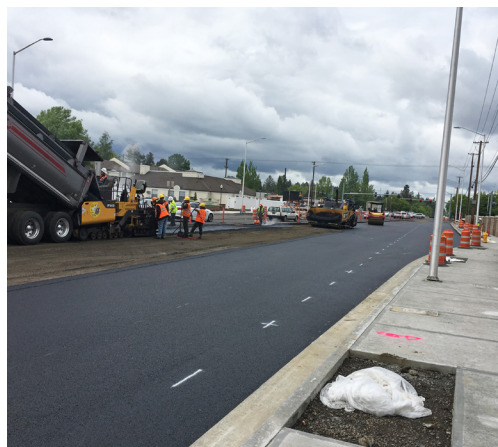
Farmington Road Improvements Award-Winning Project for Urban Arterial Paving Excellence
